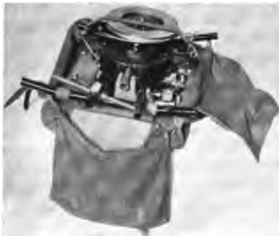
FIG. 157 b .—Generating plant of knapsack set (packed for transport). [See p. 321.]
